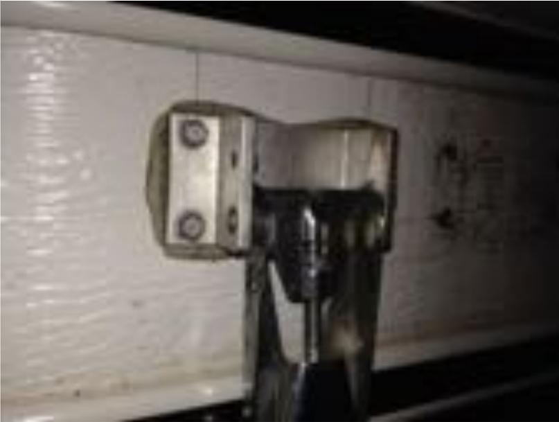
step seven: attach the offset ball bracket using 2" self tapping #10 screws by placing it up against the clip. It should be placed so the holes should line up with all the screws that attach the roof to the trim.
