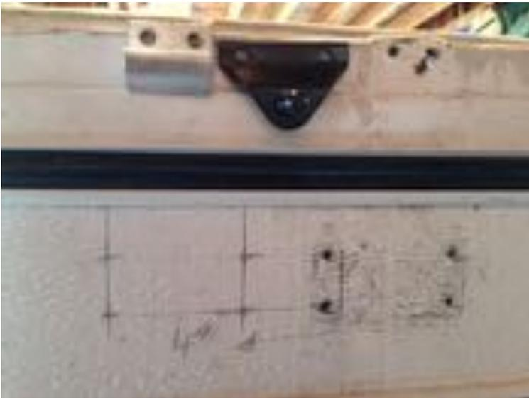
Step eight: Wouldn't you know it, the rear awning lip edge on roof is 2" too long on either end. Use a hack saw to cut these off and then a file to smooth the edges.
