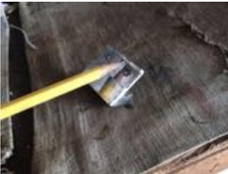
step two: The roof edge screw has to be moved from where you will put the clip so the hole under the clip just removed can be filled with that screw (always put silicone on the treads). The 2 holes left from moving the clip and the buckles can be filled with a great product... JB Weld "Water Weld" , it works and it is white
