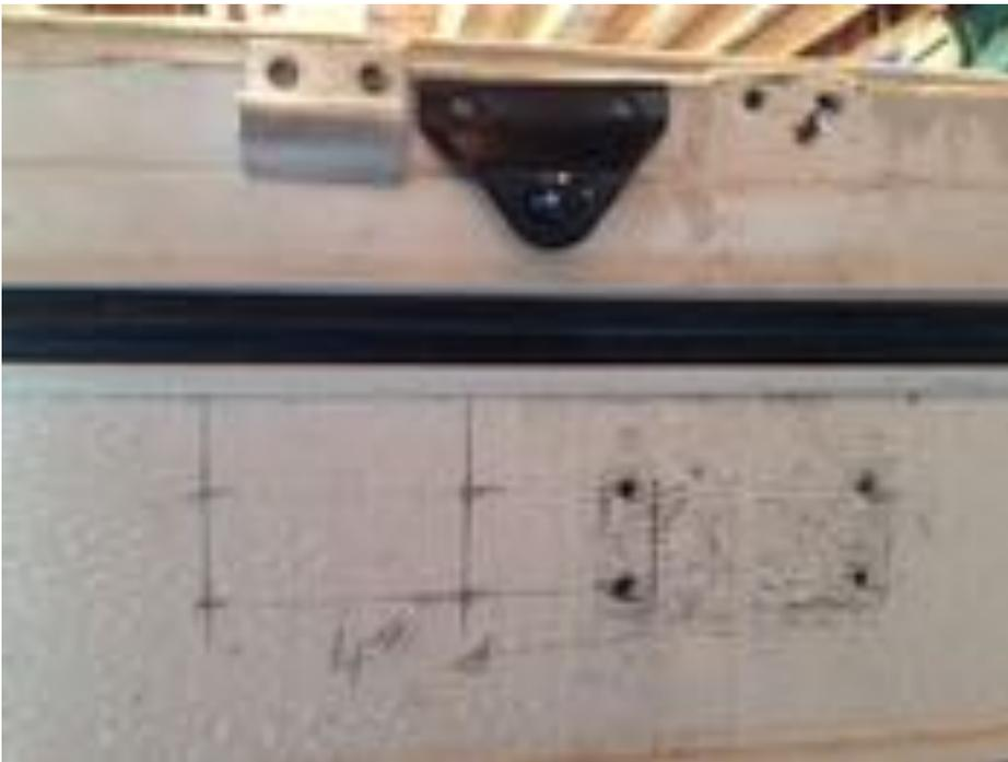
Step four: using a 3/32" drill bit make holes and then using a #8 self tapping screw, go in on all holes.
