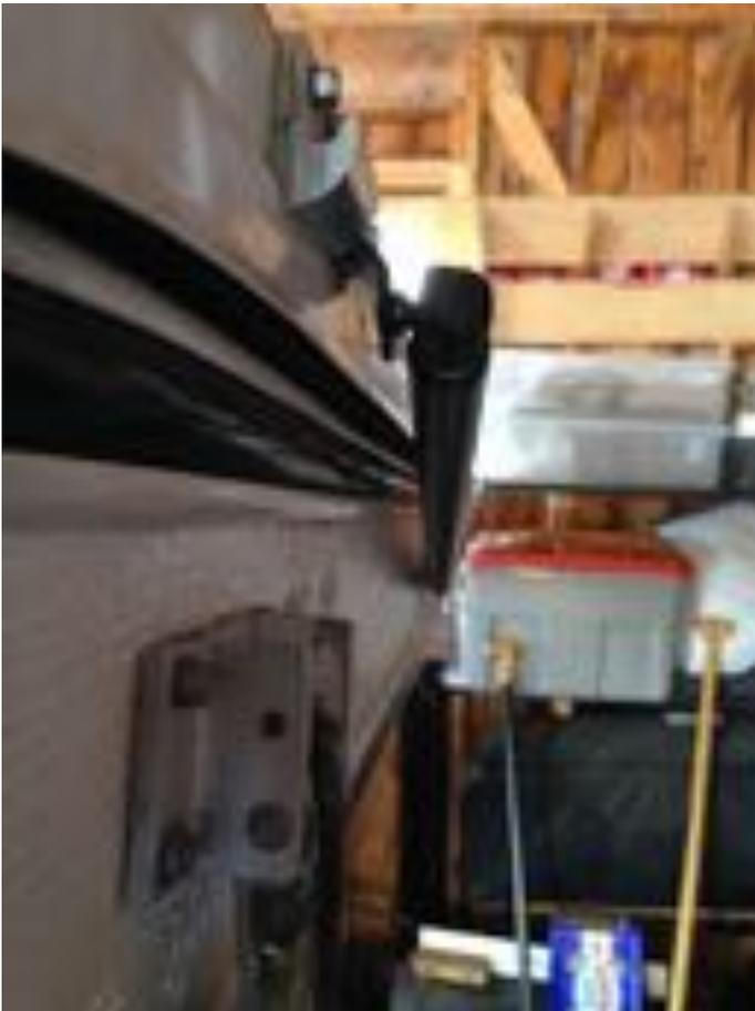
Final stage in last 2 photos: I installed aluminum plates to kick out the struts a 1/4" as well as insuring a more robust stress distribution.
